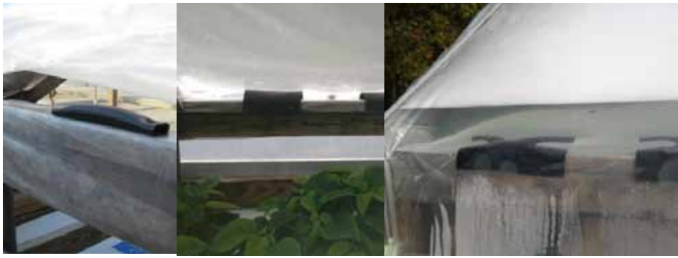
Fig. 5. Device for preventing fluid pooling at the edge of the greenhouse (left to right); black tube attached to hip frame of greenhouse, EPDM plastic covering tube; pooling of the soap solution that continued to occur.
