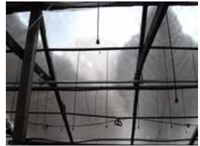
Fig. 1. Bubble system in operation, filling the void with soap bubbles.
