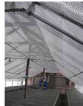
Fig. 2. Thermal curtain after installation.
