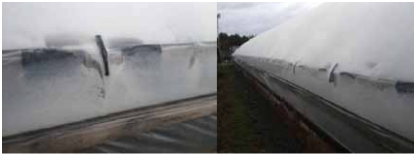
Fig. 6. Black tubing placed vertically between the two layers of plastic, which effectively eliminated the pooling problem.
